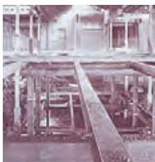
The existing superstructure has been retained
