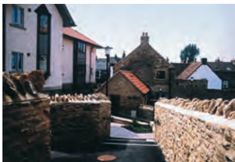
The Guinness Trust and Knightstone Housing Association have combined in Frome, Somerset, to create 'The Piggeries' – a mix of high density housing that responds sensitively to local context
