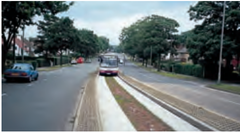
Dedicated busway, Leeds
