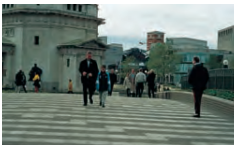
With part of the road lowered and a wide pedestrian crossing provided, an area once severed now binds together seamlessly
