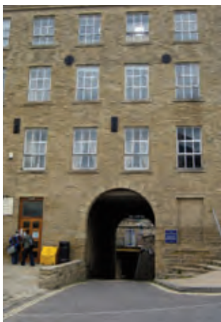
Mill buildings have been converted into a mix of offices and high quality flats
