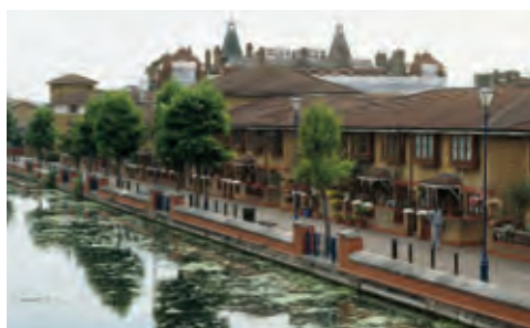
The lack of forecourt parking ensures building thresholds are not dominated by cars
