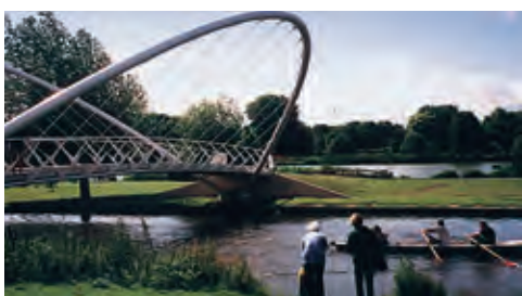
Ouse Bridge, Bedford (Architect: Chris Wilkinson)
