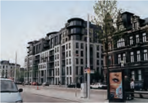
A modern perimeter block in Antwerp, Belgium, that responds to the scale and rhythms of adjacent buildings
